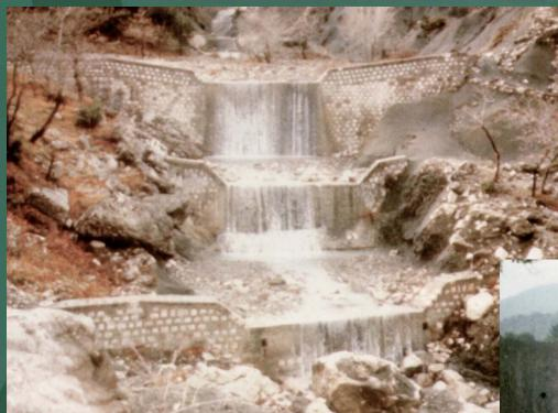
Dam for consolidation of the river bed in a Mt. Pindos torrent
